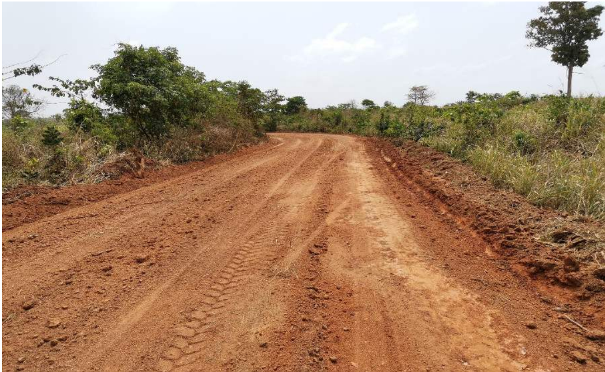
Plate 3: Road maintenance/construction in Miremano
