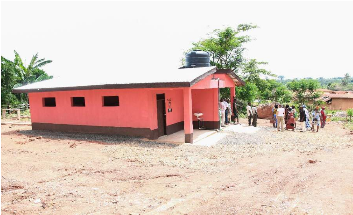
Plate 1: Ablution facility in Kotaa community
